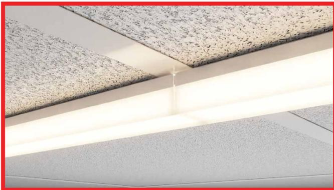
\*\*\*Important Note for installing connected fixtures: Join the two sections by pushing the them together. Ensure to keep the two sections aligned while joining to so the joining tongue engages with the channel on the back side of the fixture. Reference shop drawings for driver locations and low voltage whip routing.
